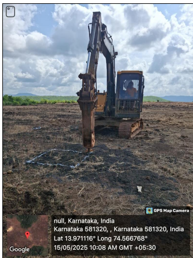
Fig 6.8: Pitting work being attempted in the Field.
